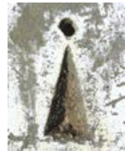
Drill Hole and Wing in Kerb
