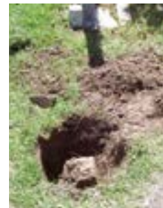
Concrete Block and Boundary Peg
